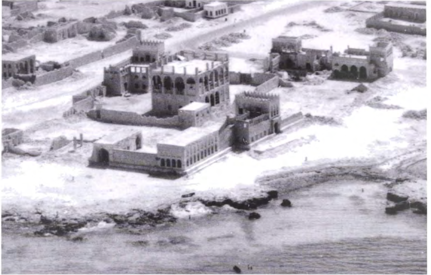
(Fig. 1) : A General View of the Old Palace before restoration.
